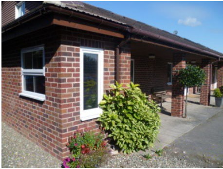
Covered walkway access to front doors to all Cottages from the car park
